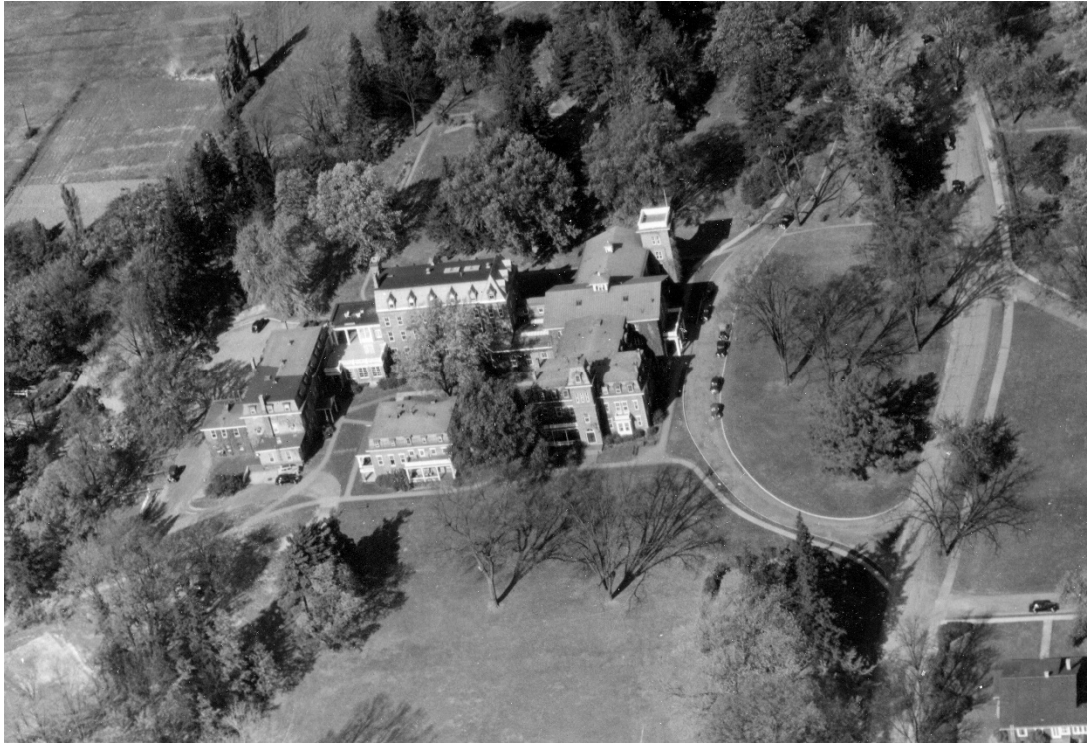
An aerial view of the Mansion House and environs, ca. 1940. (OCMH Collection)
