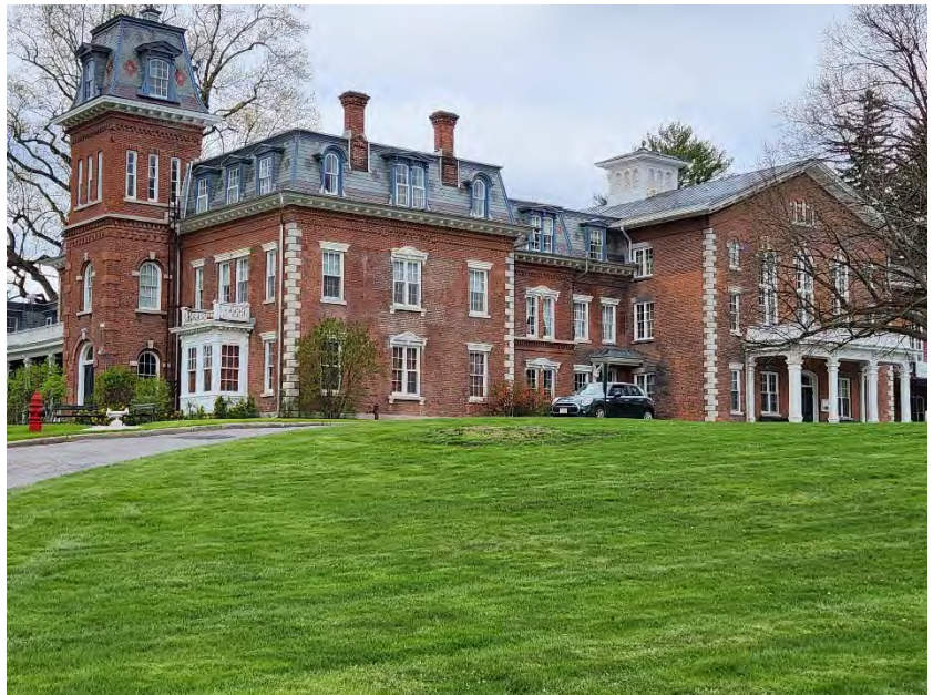
Currently the Mansion House is inaccessible to persons with disabilities; each of the building's entrances must be accessed via steps or stairs.
