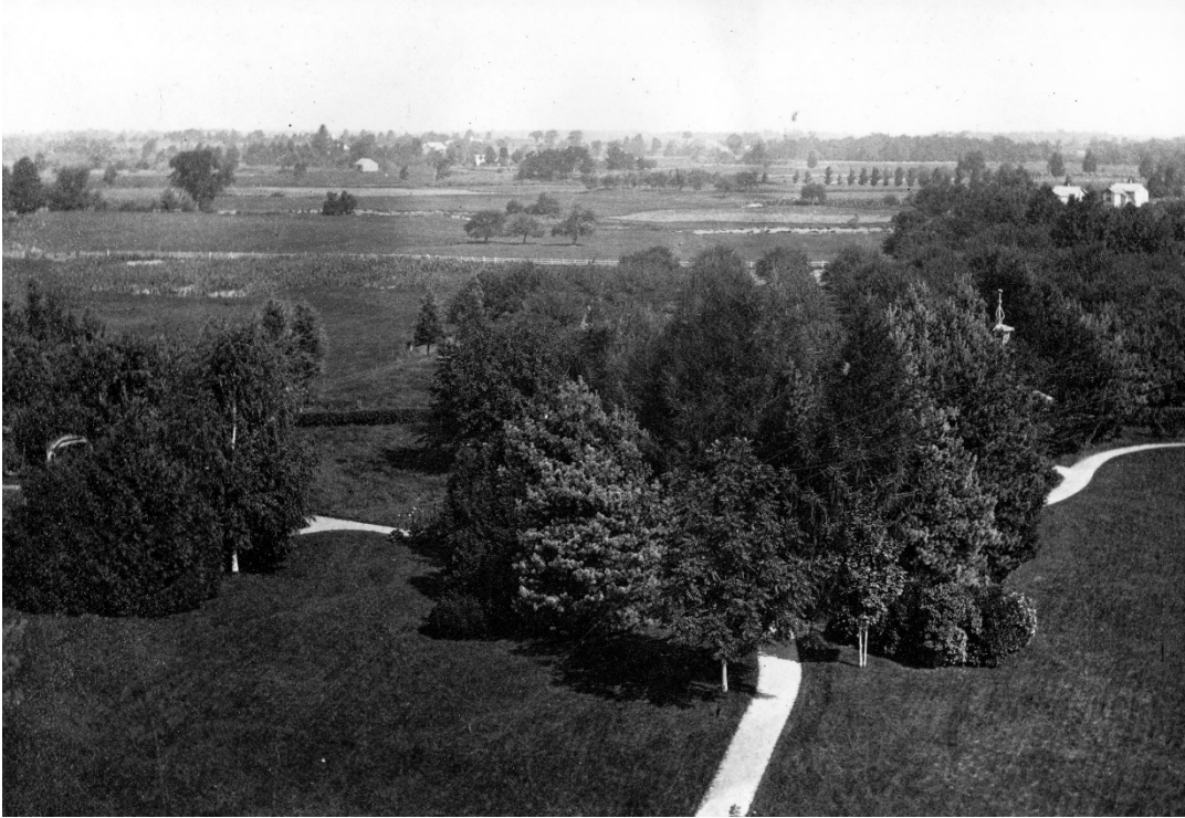
1874. View over North Lawn with perimeter pathway taken from north tower
