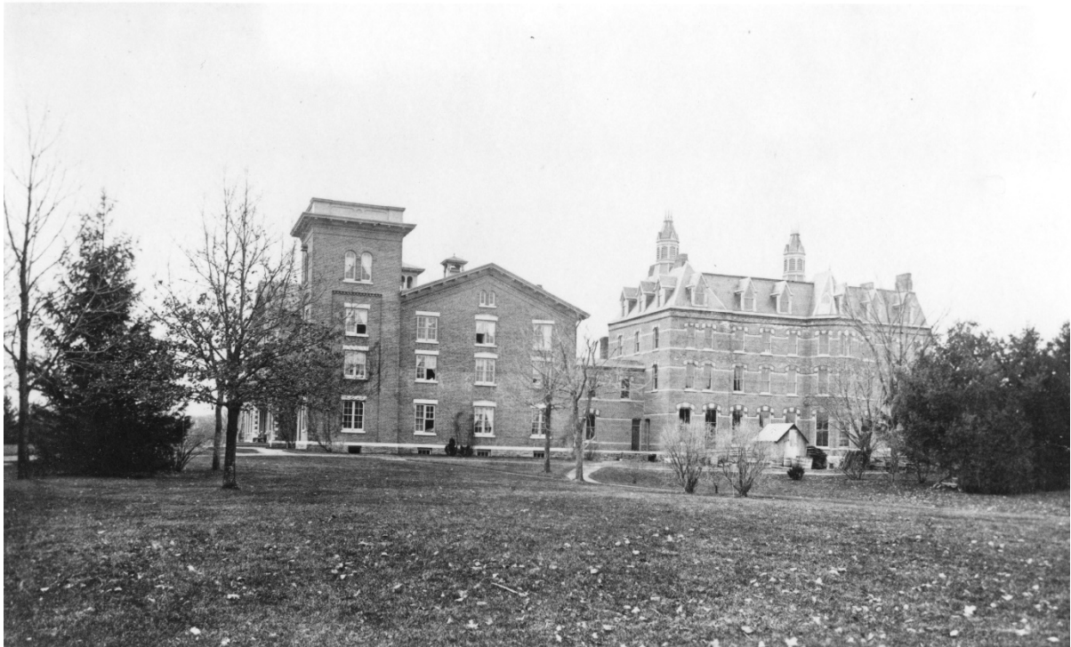
1878. Mansion House (and New House) looking across the North Lawn, southward
