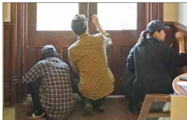
After a tutorial in conservation treatment and color-matching, Cornell students get to work in-filling all the areas of damage on the interior woodwork.
