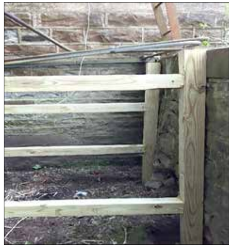
Temporary shoring of the retaining wall
