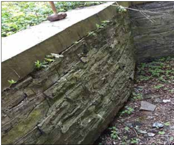
Southward deflection of the retaining wall showing it in a stage of imminent collapse
