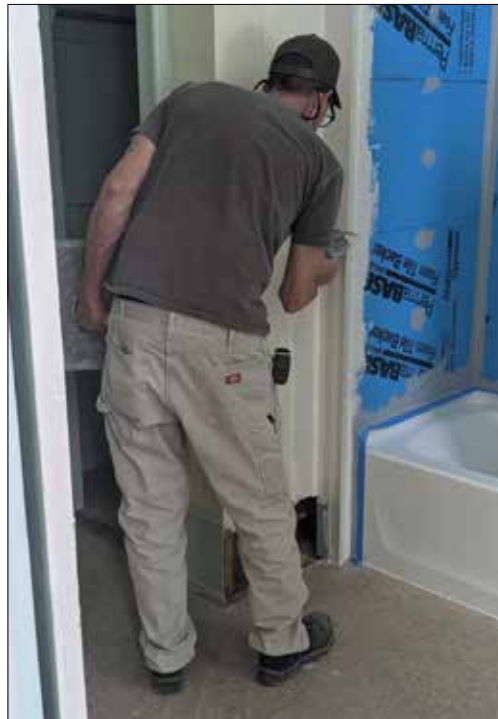
Employee Chris Stedman working on a guest bathroom
