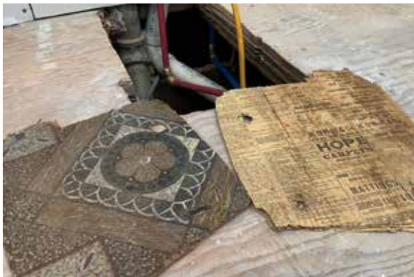
Remnants of an 1892 newspaper were found when cutting into the floor of this bathroom for plumbing
