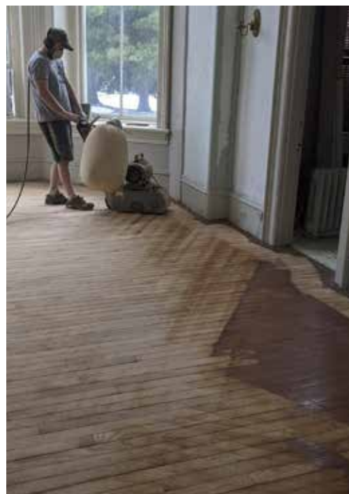
Clinton Hardwood Flooring sanding the floors for refinishing in January 2021
