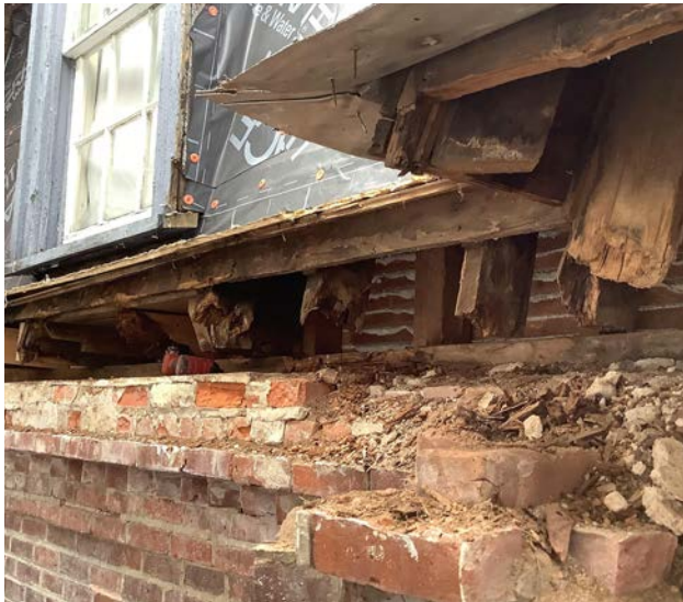
Before: Water damaged the bricks and mortar, deteriorated the wood framing and cornice; Cornice was repaired and replaced with mahogany
