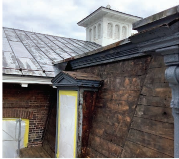
Slate removal, South Wing Quad – 9/21
