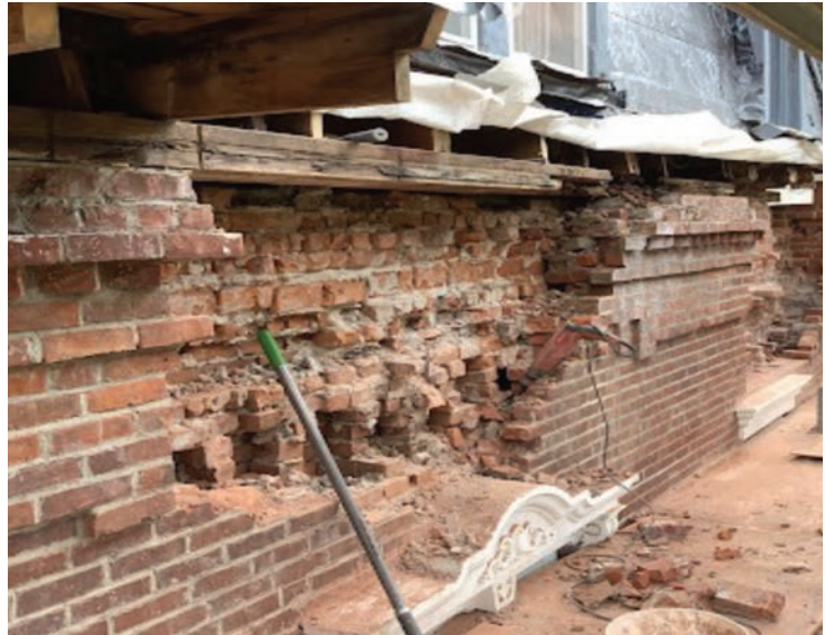
Brick facade rehabilitation, South Wing and East elevations – 6/22-8/22
