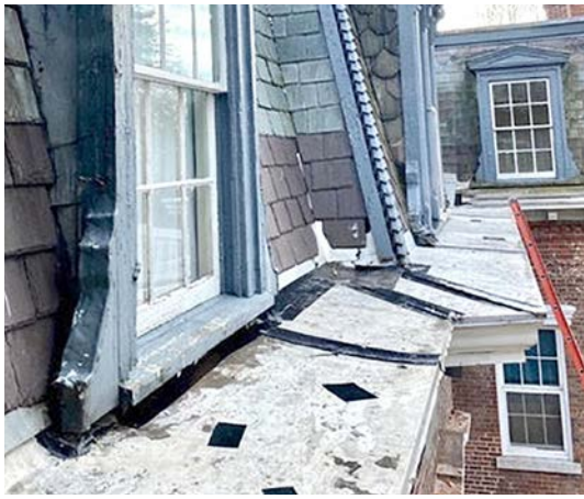
Before: Water damaged the bricks and mortar, deteriorated the wood framing and cornice; Cornice was repaired and replaced with mahogany
