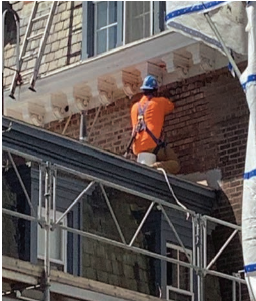
South Wing Masonry repointing – 4/22
