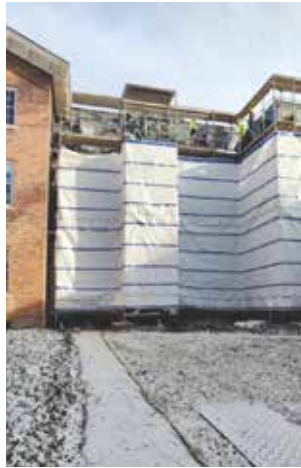
Enclosing the scaffolding for work to commence
