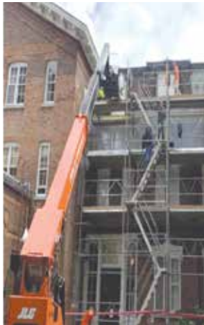
Contractors prepping for demo on the mansard roof
