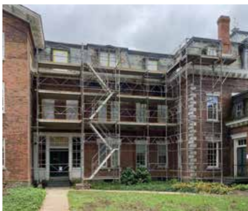
After the construction of the bridge was complete, mobilization would soon be underway, and four stories of scaffolding were brought in and erected
