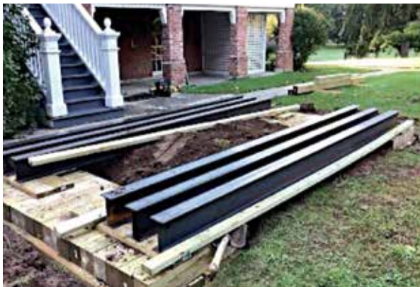
Structural engineering firm Ryan Biggs Clarke Davis was brought in to design this specialty access bridge, which would need to include a weight capacity rating able to handle up to 30,000 pounds
