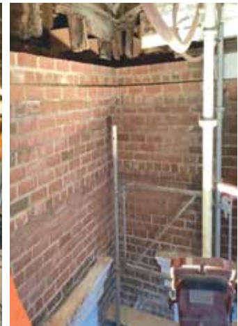
Left side tied into the 1862 Building
