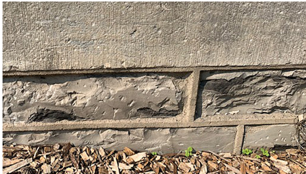
Close-up of the mortar work mentioned above
