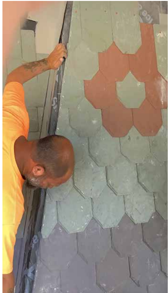
Replacement of deteriorated slates and trim (Preservation)
