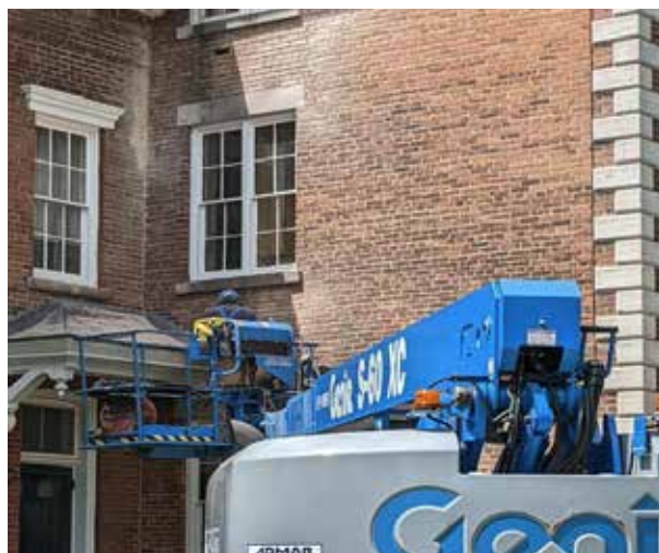
Intersection of the 1862 Building and the South Wing, East Elevation
